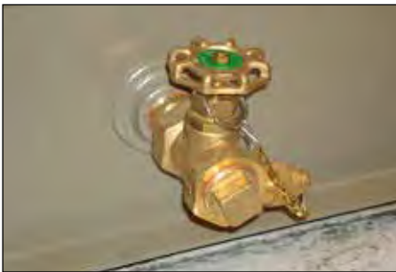
Figure 3. Drain valve with sampler.
