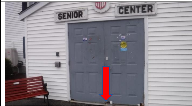
Front doors rust, corrosion, hole, duct tape
