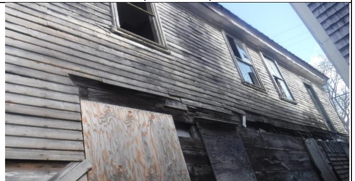
Missing siding, broken windows
