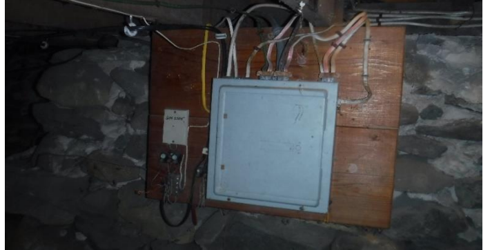
Old circuit breaker panel and wiring
