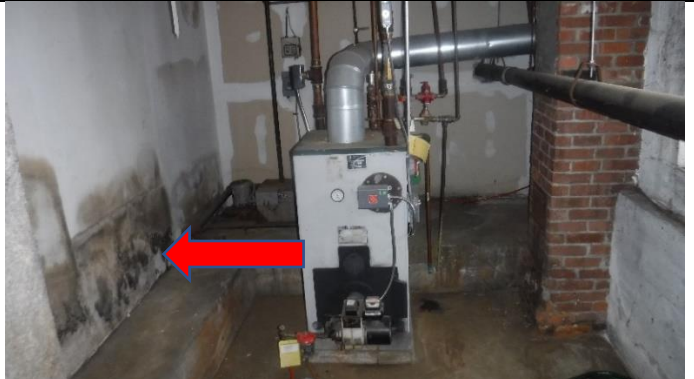
Oil furnace with Becket burner, possible mold on wall
