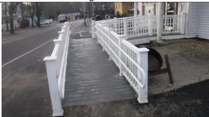
Front Entrance handicap ramp needs antiskid paint
