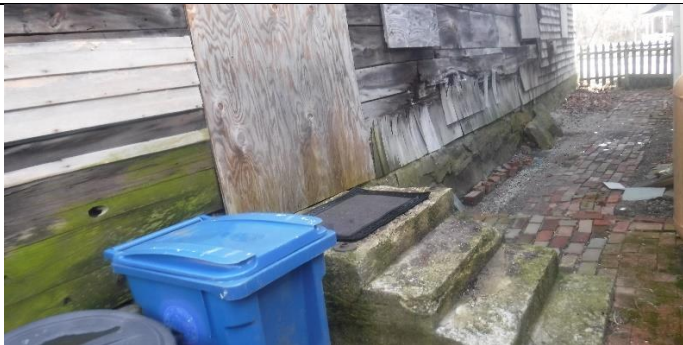
Boarded up side door, old damaged steps
