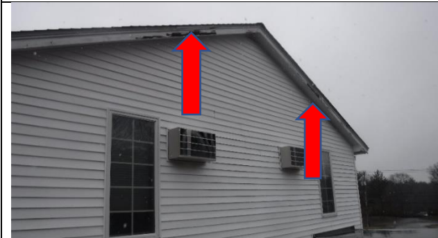
Rake edge peeling paint, rot, close up
