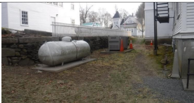
Propane tank and generator
