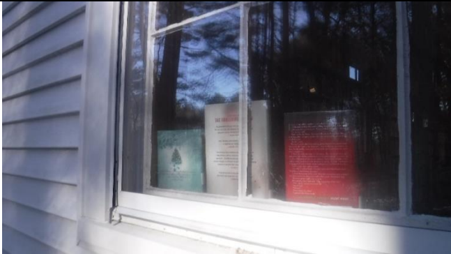
Storm window over single pane glass
