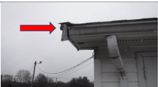
Northwest corner rake edge decay
