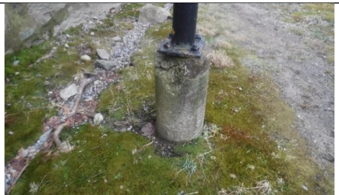
Fire escape round concrete support in disrepair
