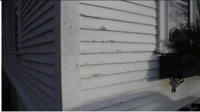
Wood clap board siding paint peeling
