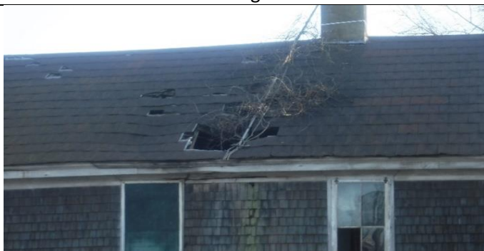
Large hole in roof
