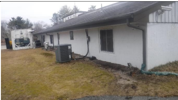
South side buried in soil piled high
