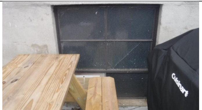
Oil burner room cracked window
