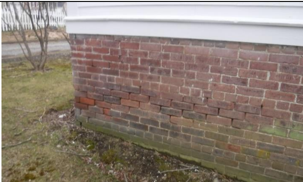
Rear of building bricks need repointing
