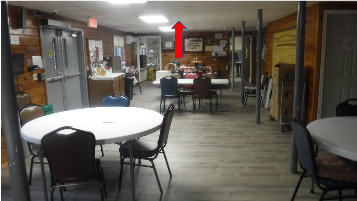
1 st Floor small activity area ceiling grid sagging in some areas
