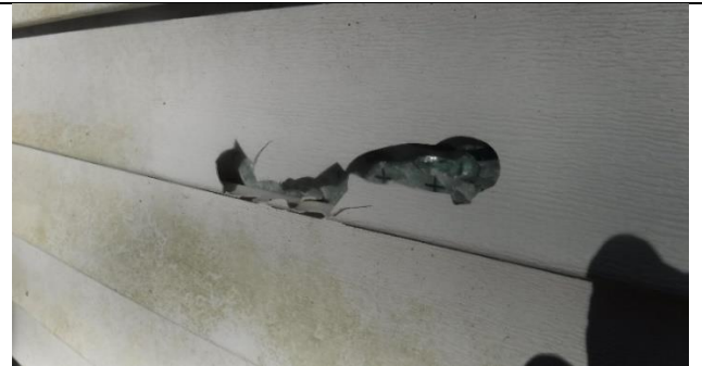
Close up of damaged siding, mold, mildew
