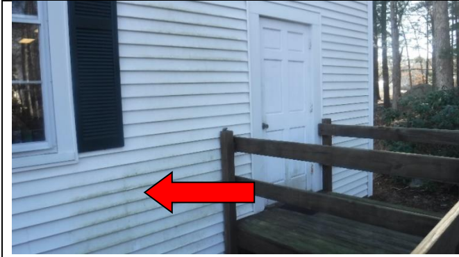
Side handicap entrance, mold on vinyl siding
