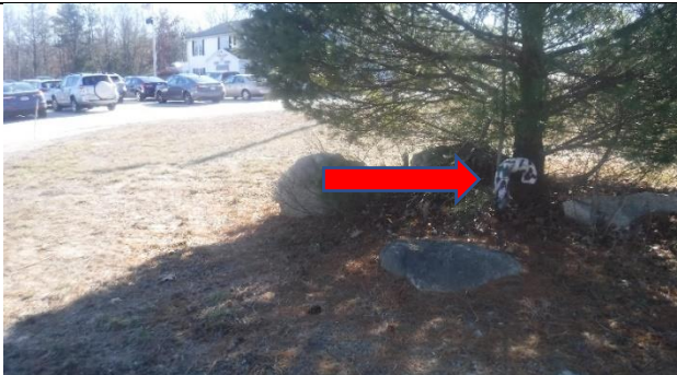
Leaching field vent pipe
