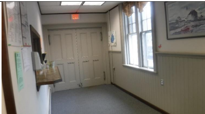
Second Floor doors to first floor exit ADA non-compliant
