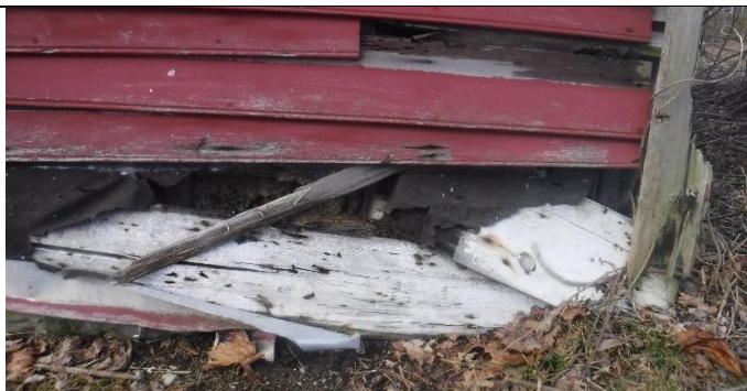
Insect damage to wood
