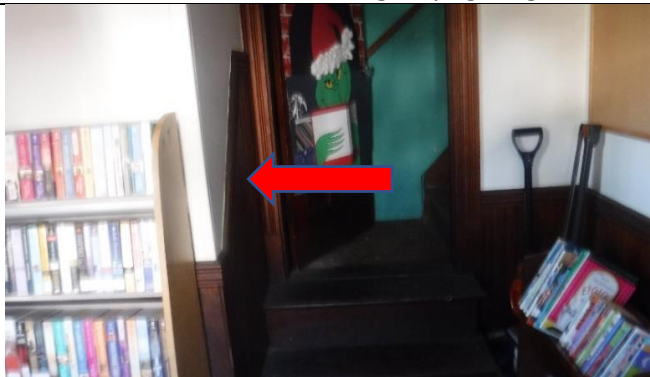
Stairs to attic no railing
