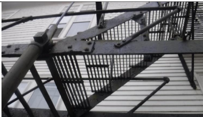
Corroded untested fire escape
