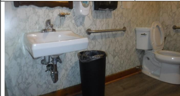
1 st Floor rest room 2 sink ADA non-compliant
