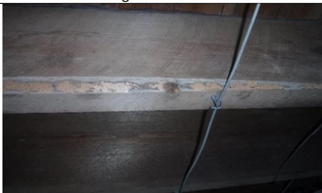
Evidence of powder post beetles close up view
