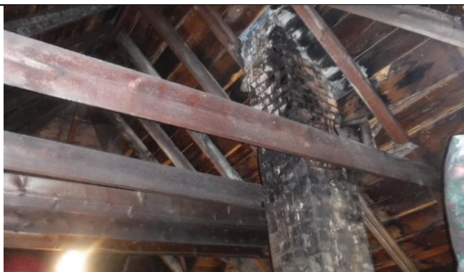
Old roof leaks around chimney
