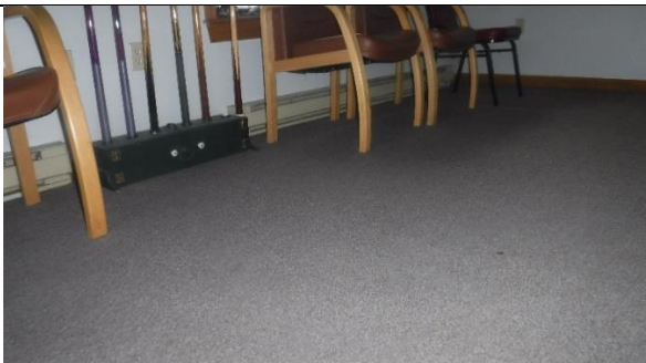
Base board electric heat
