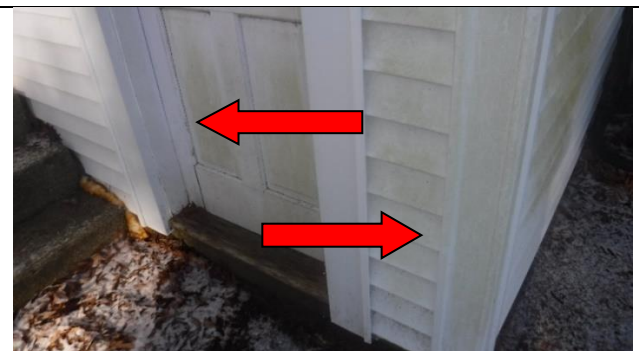
Door splitting, unpainted threshold, mold on siding
