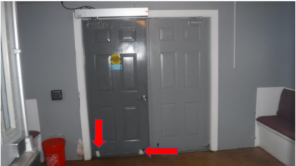
Handicap Double Doors rusted, rotted, holes, duct taped
