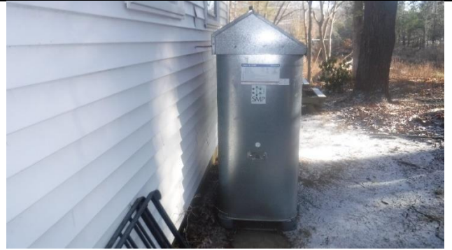
Outdoor double wall oil tank
