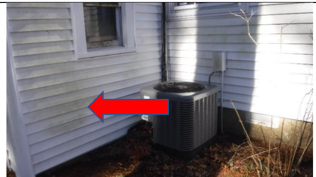
Air conditioner compressor, mold on siding
