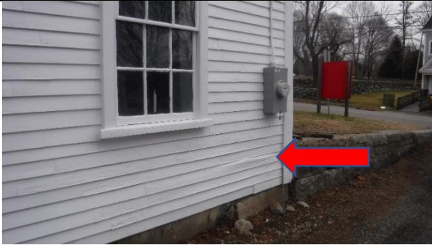
Siding protrusion
