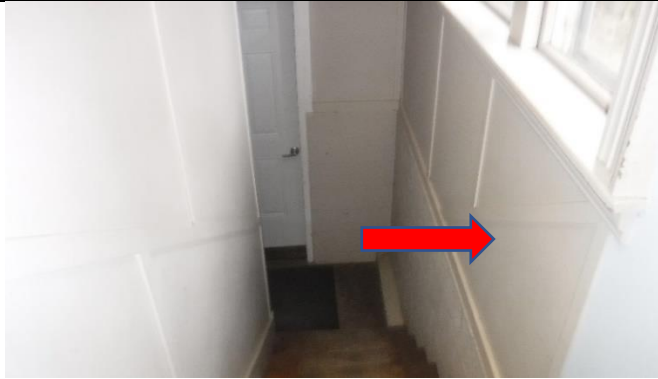
Narrow staircase to basement, no railings, suspect ACM panels
