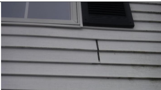
Gap in vinyl siding close up
