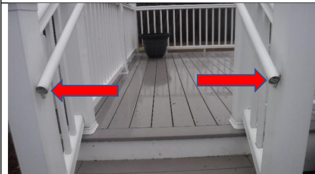
Missing railing caps - sharp edges
