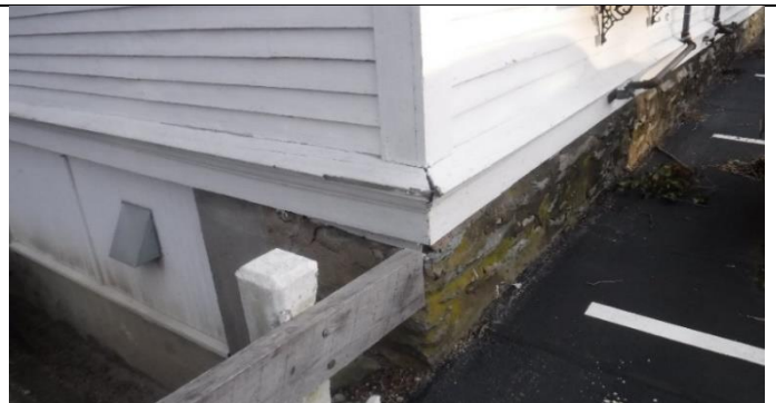
Mitered corner wood decaying
