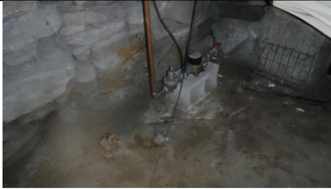
Water main damp exposed soils floor area
