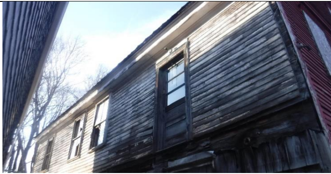
Broken windows, rotting, insect damaged wood
