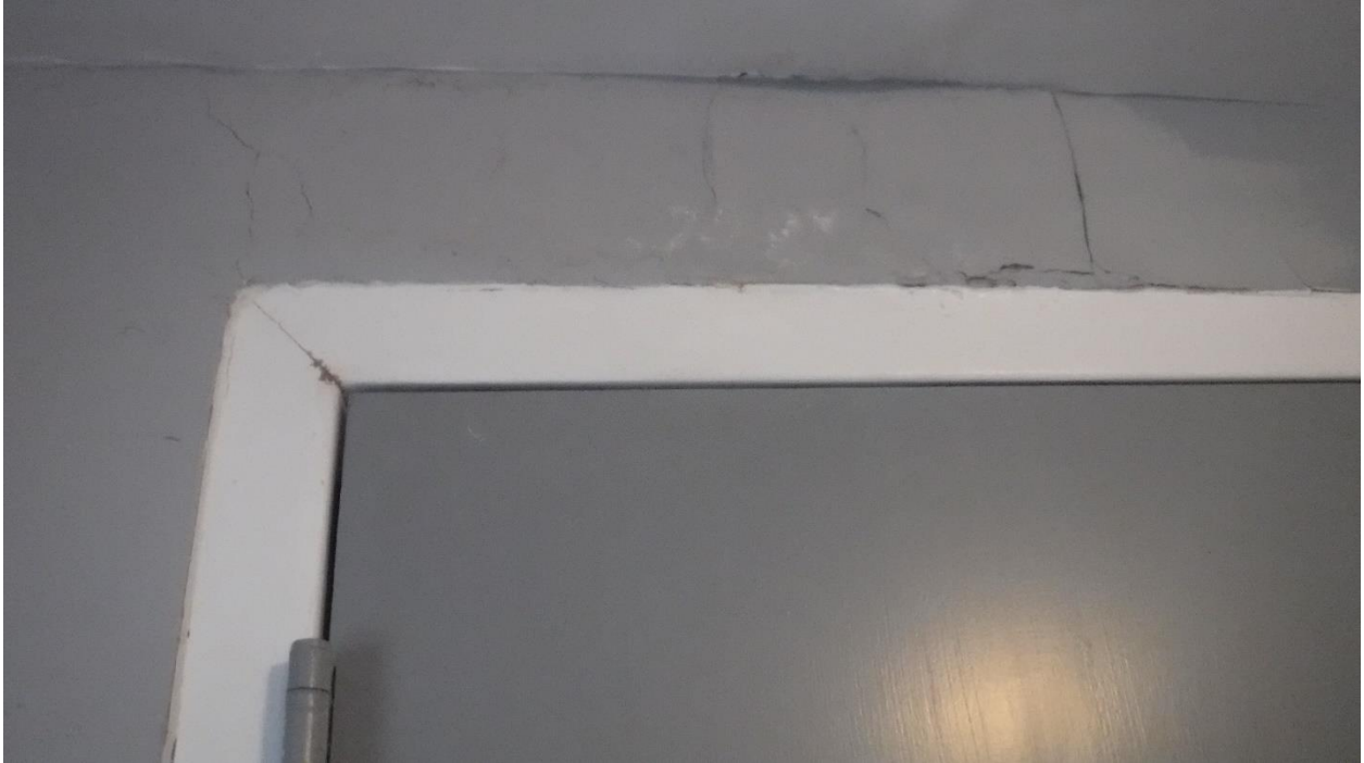
Vestibule drywall water damage
