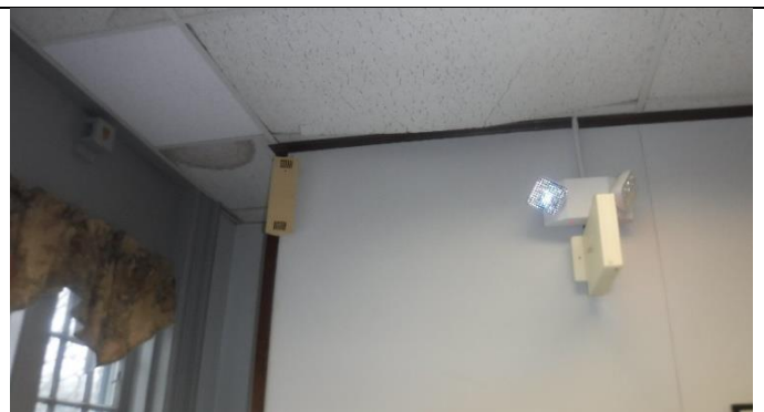
Damaged leaking, sagging ceiling
