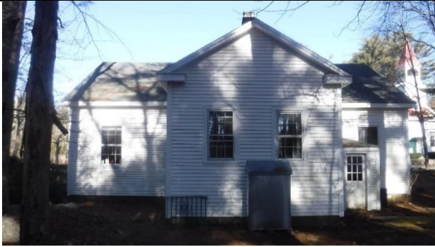
Rear of building, double wall oil tank
