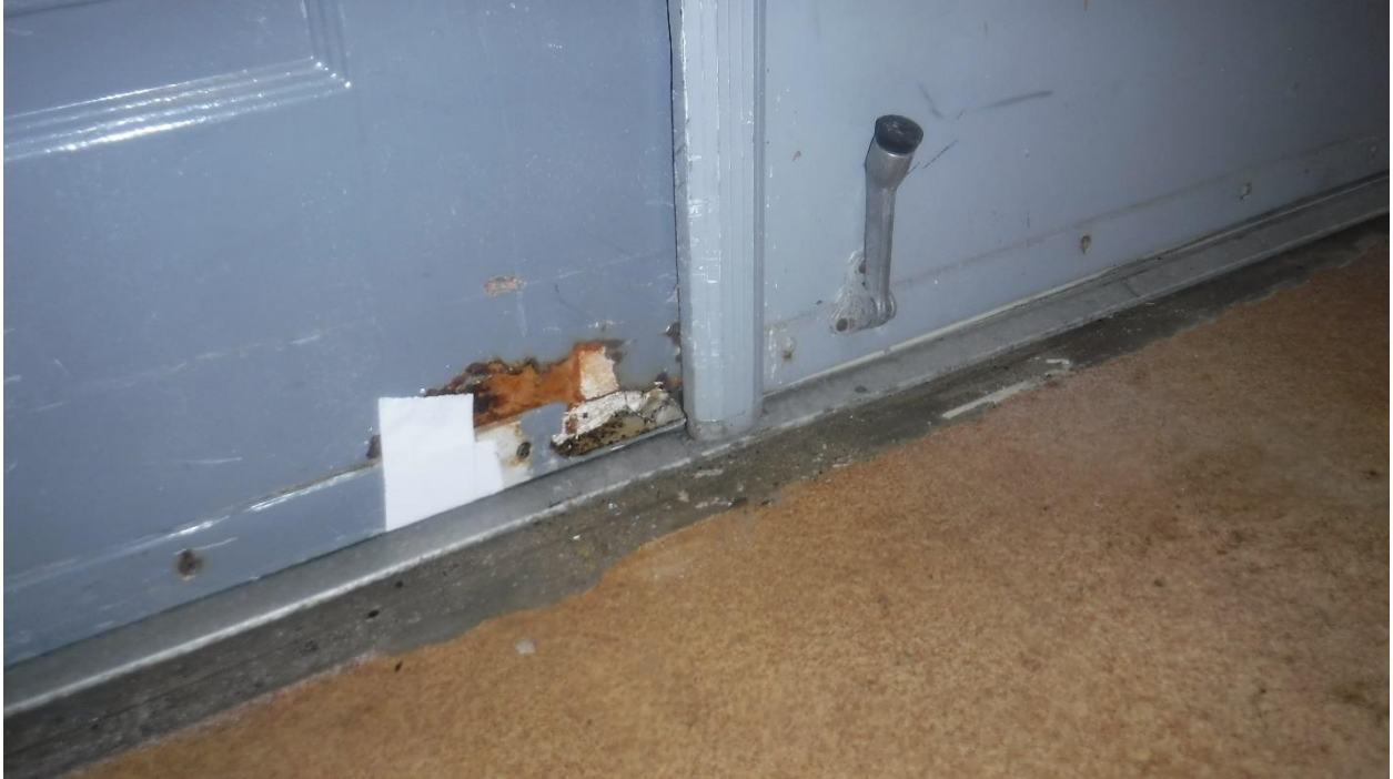
Vestibule exterior metal double doors corrosion, rusted through hole
