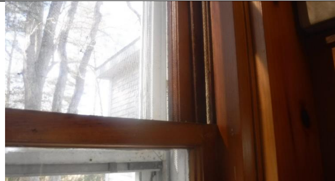
Single pane wood rope and pulley windows
