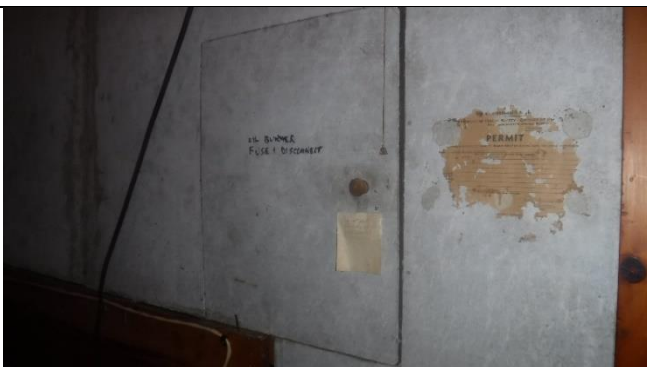
Oil burner shutoff switch behind suspect panel
