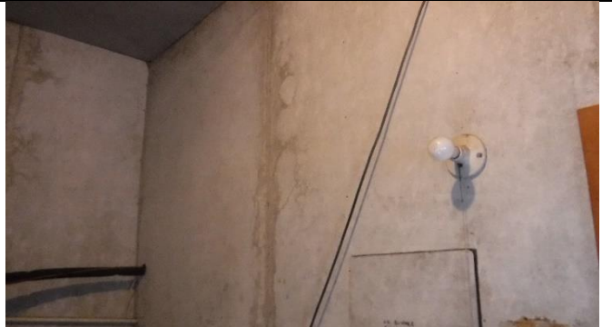
Suspected asbestos containing panels, walls, ceiling
