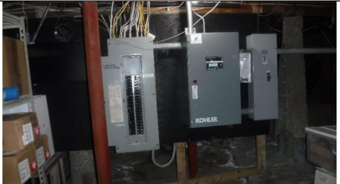
Circuit breaker and generator panels
