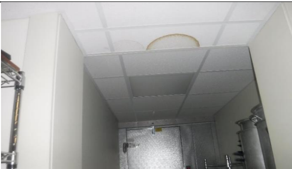
Walk-in cooler and freezer ceiling leak
