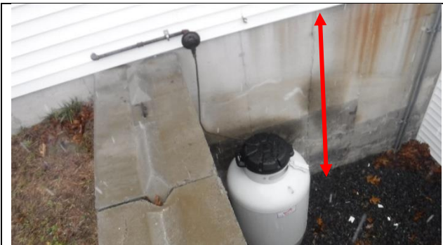
Propane tank against building and 9 foot drop
