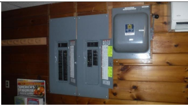
Circuit breaker panels and manual generator switch
