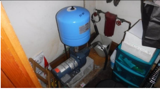
Well pump and expansion tank
