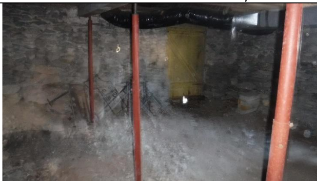
Steel jack support building structure - exposed soils floor
