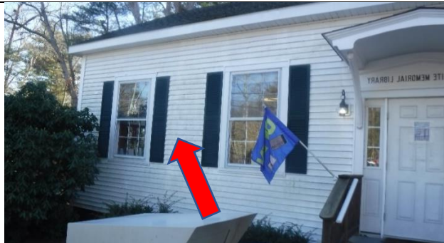
Left front mold, mildew on vinyl siding
