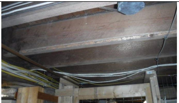
Floor joist with evidence of powder post beetles
