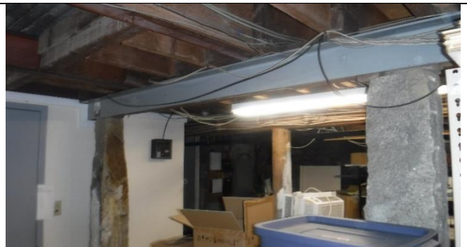
Steel girder with granite supports
