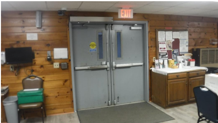
Handicap electrically operated doors to unheated vestibule
