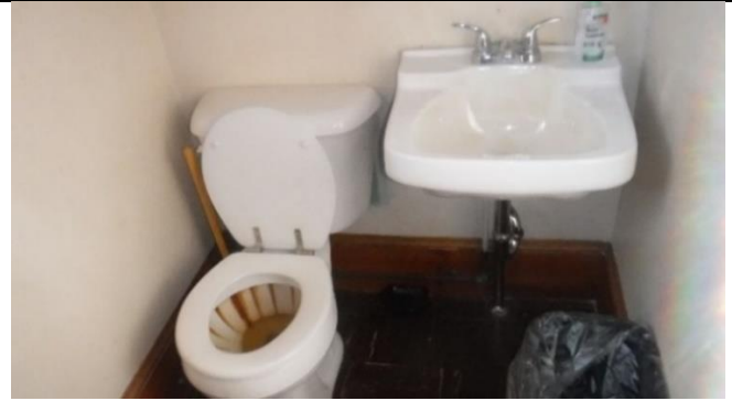
ADA non-compliant bathroom, rust in toilets
