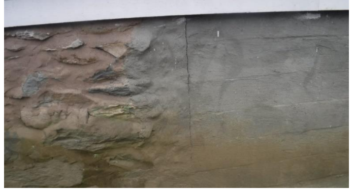
Crack in foundation close up
