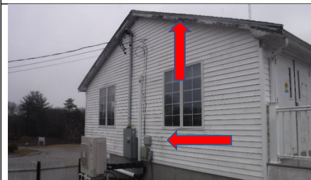
Rake edge peeling paint, rotted wood, siding mold
