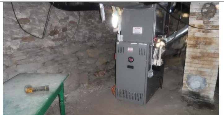
Furnace and air conditioning split system
